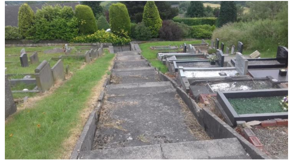
Photo 12: Top of flight of concrete steps looking down towards point C, black iron gates onto Taylor Lane 22/6/2017
